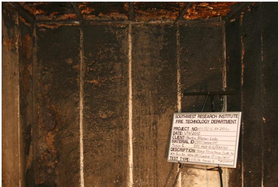
Figure 4. Post Inspection (back wall).
