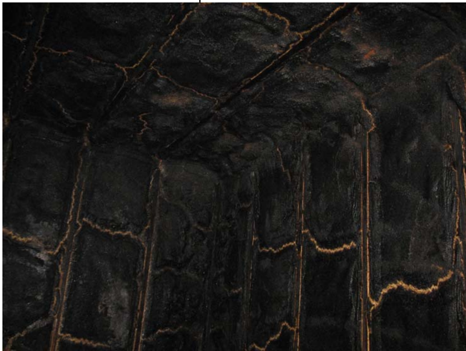
Post test picture of corner above burner
