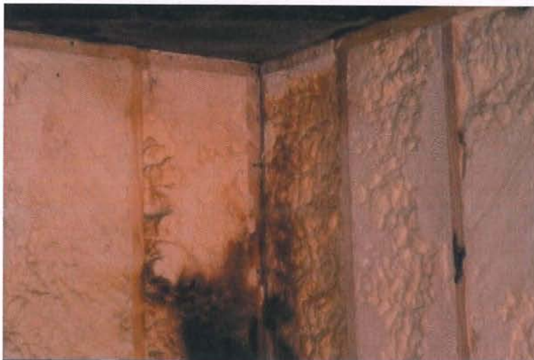
Figure 4. Post-Test: View of Burn Corner with Gypsum Removed.
